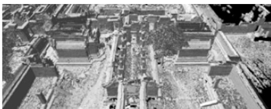
Figure 5: Point-cloud data of Gopura II.
